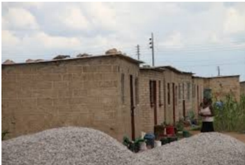
Temporary homes built for Hopley residents that have become permanent homes. Sunday Mail February 28, 2016. Picture by Tafadzwa Kadani. Pic.1
