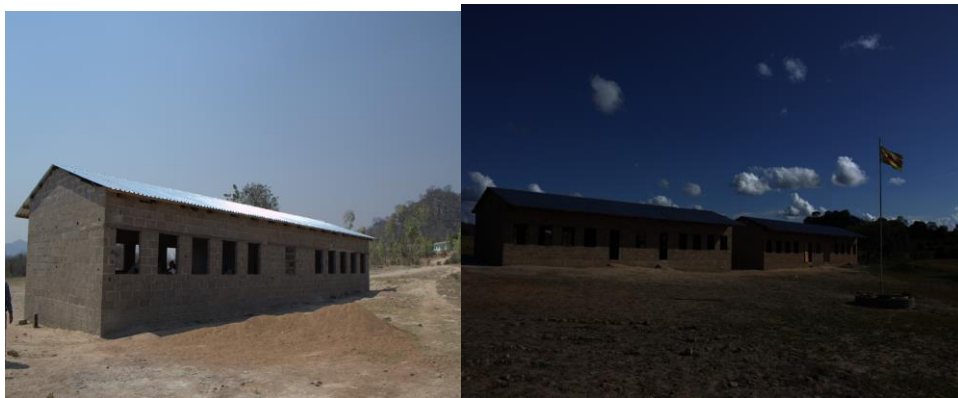
Fig 7: Zibwowa secondary school in ward 20. Image source: ECLF 2016
