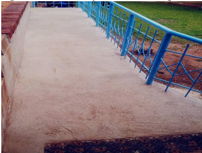
Figure 4.1 shows newly constructed ramp at Zvishavane campus
