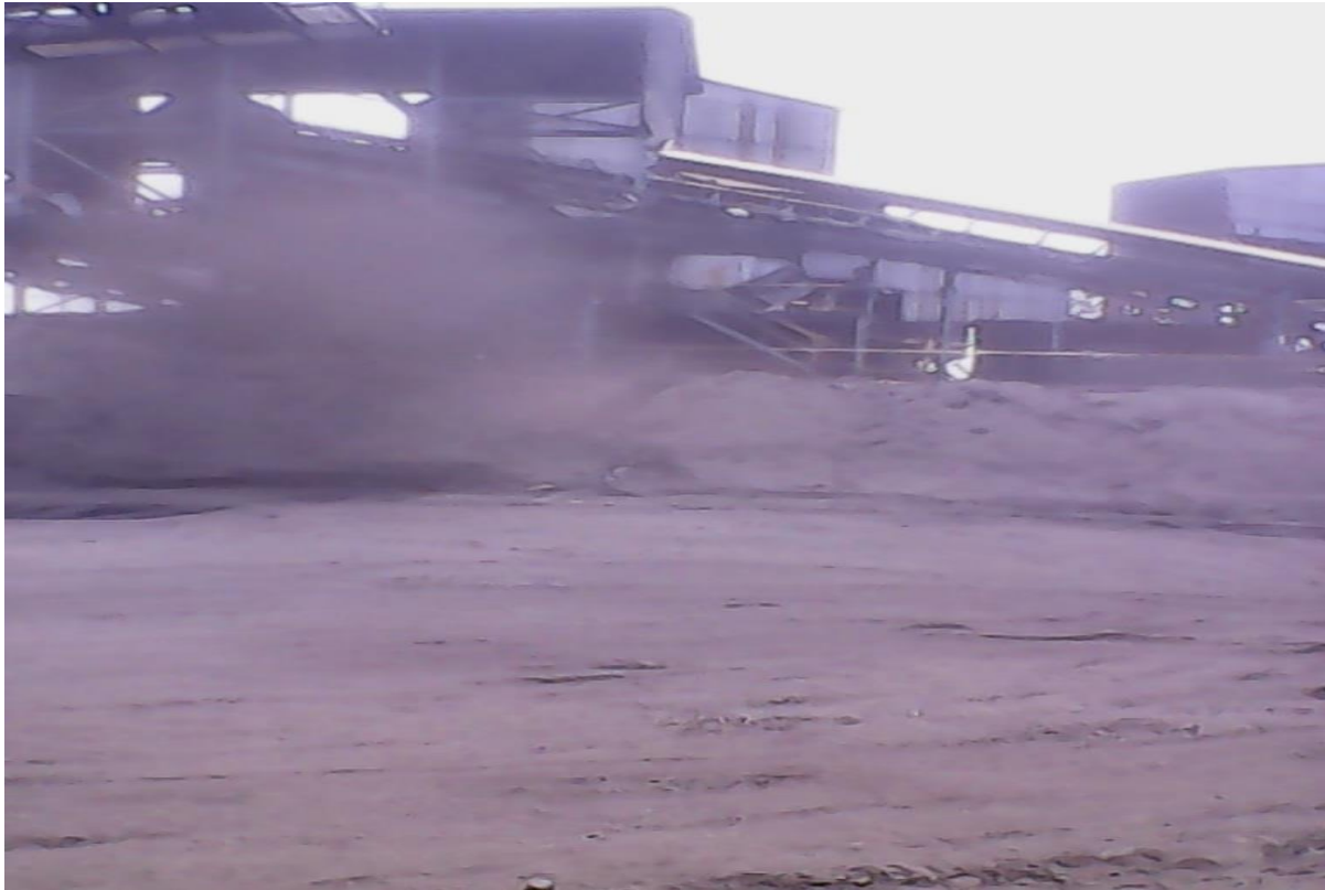
Plate 4.1: High Dust Levels at the Crushing Station
