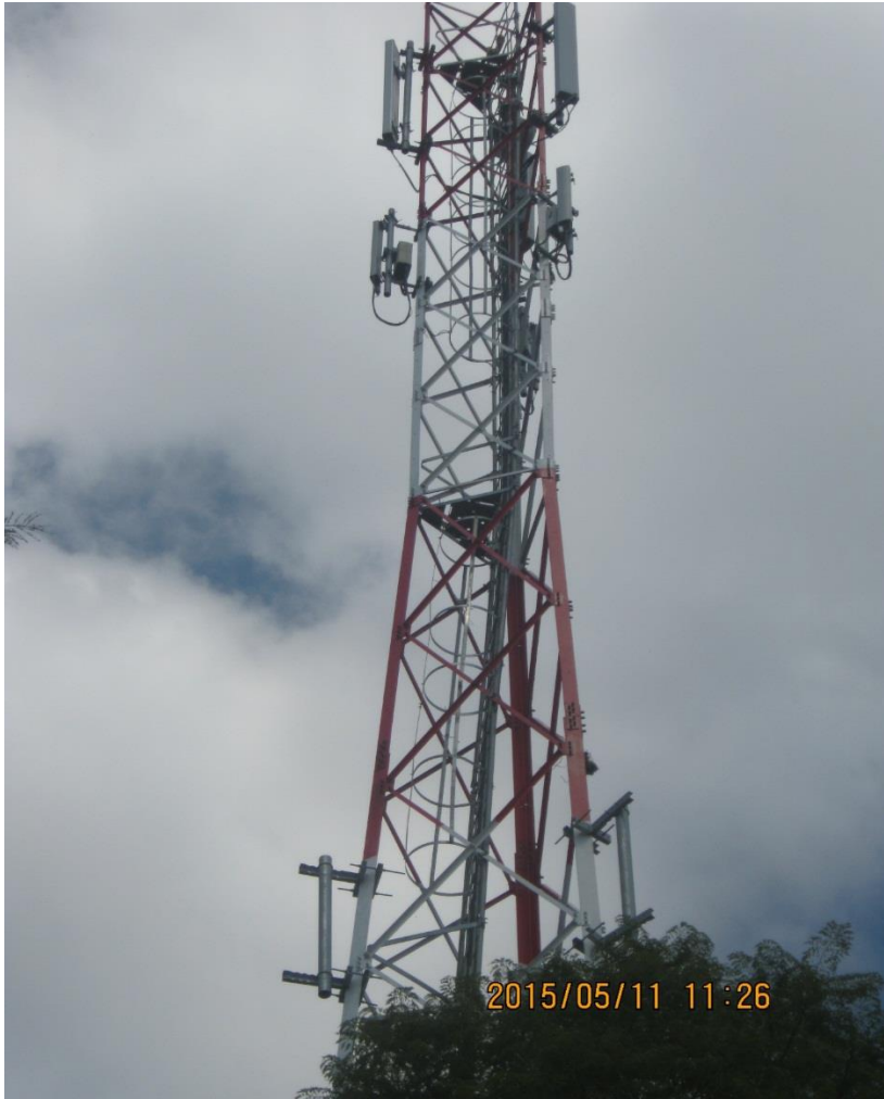
Figure 3.3 Mobile base station with 3G (2100MHz) antennas at the bottom and dual band (900MHz and 1800MHz) at the top.
