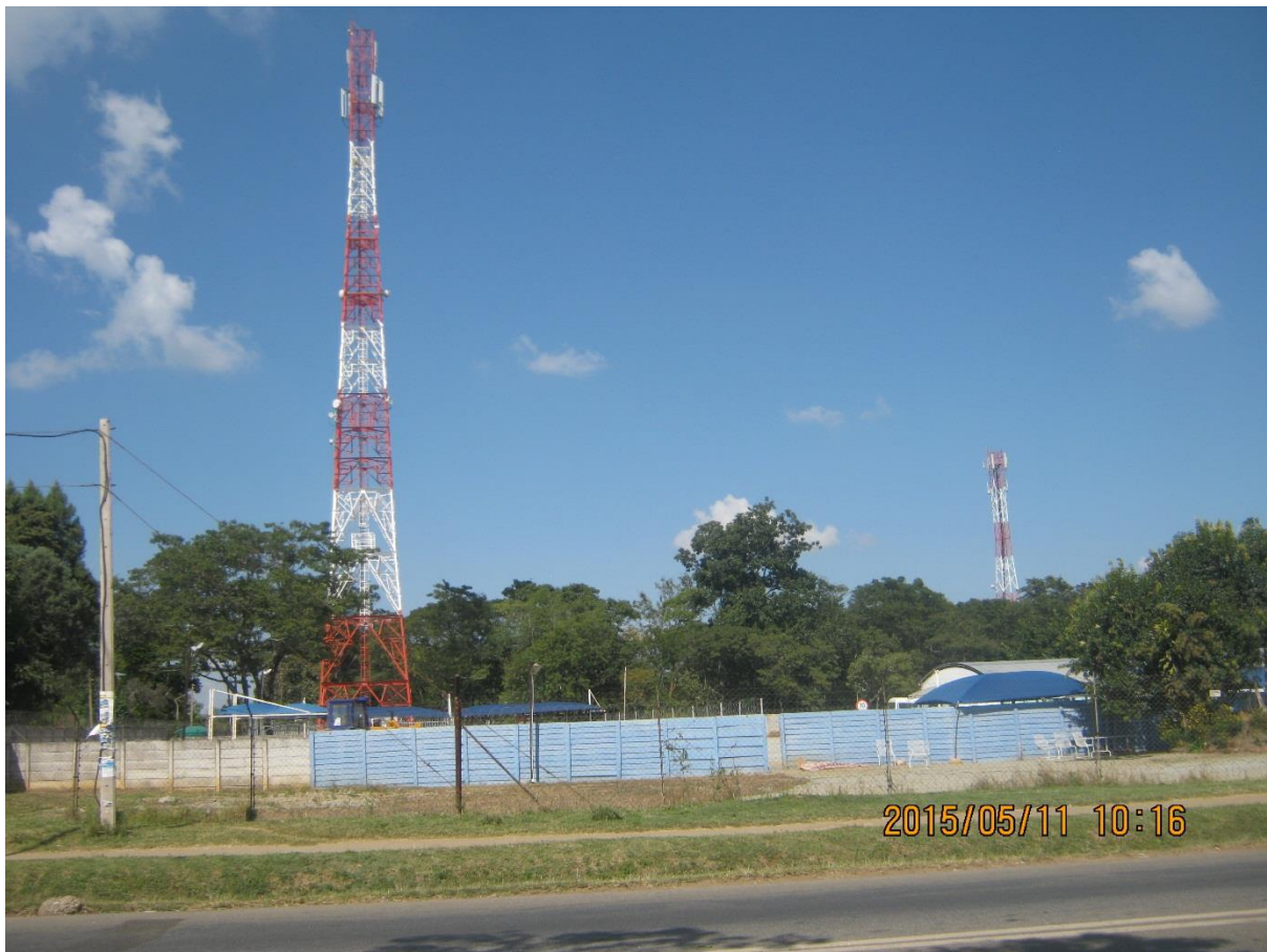
Figure 2.16 Two cellular base stations in proximity near Greencroft Shops, Harare, Zimbabwe.
