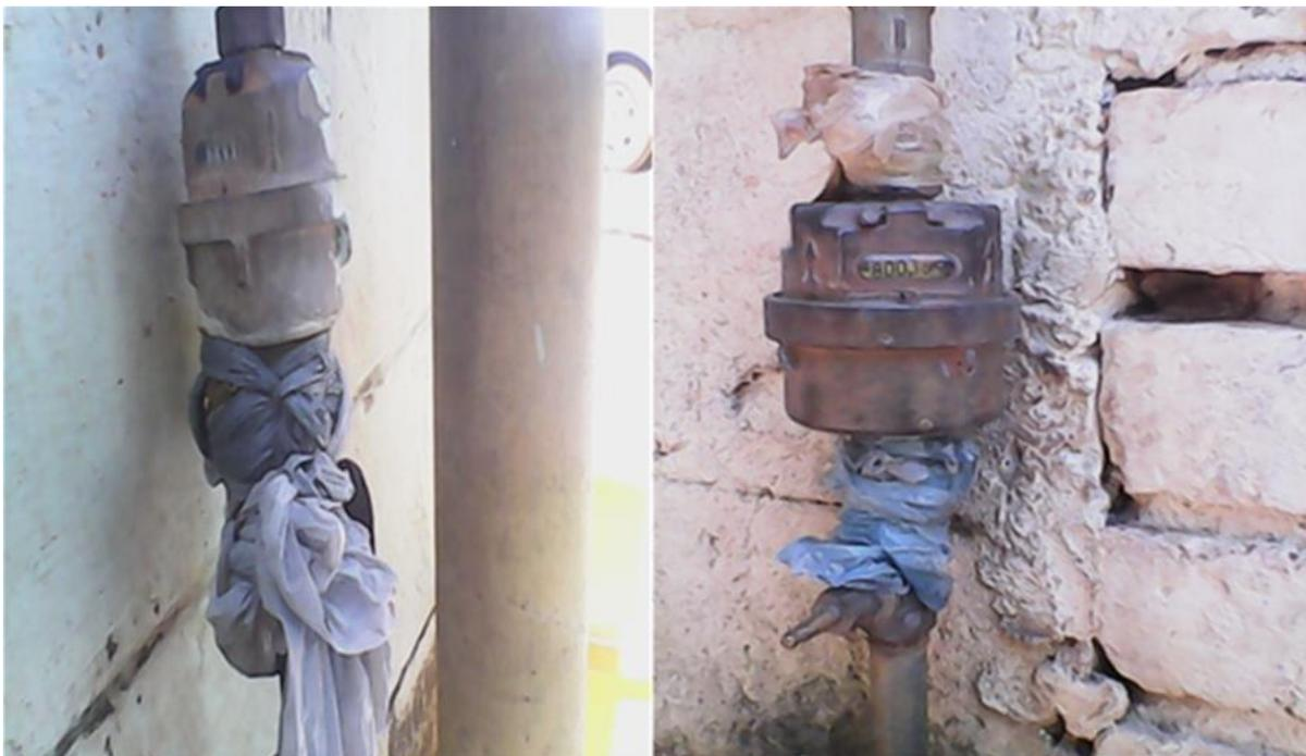
Plate 2: Two sealed leakages identified on meters in Makusha residential suburb
