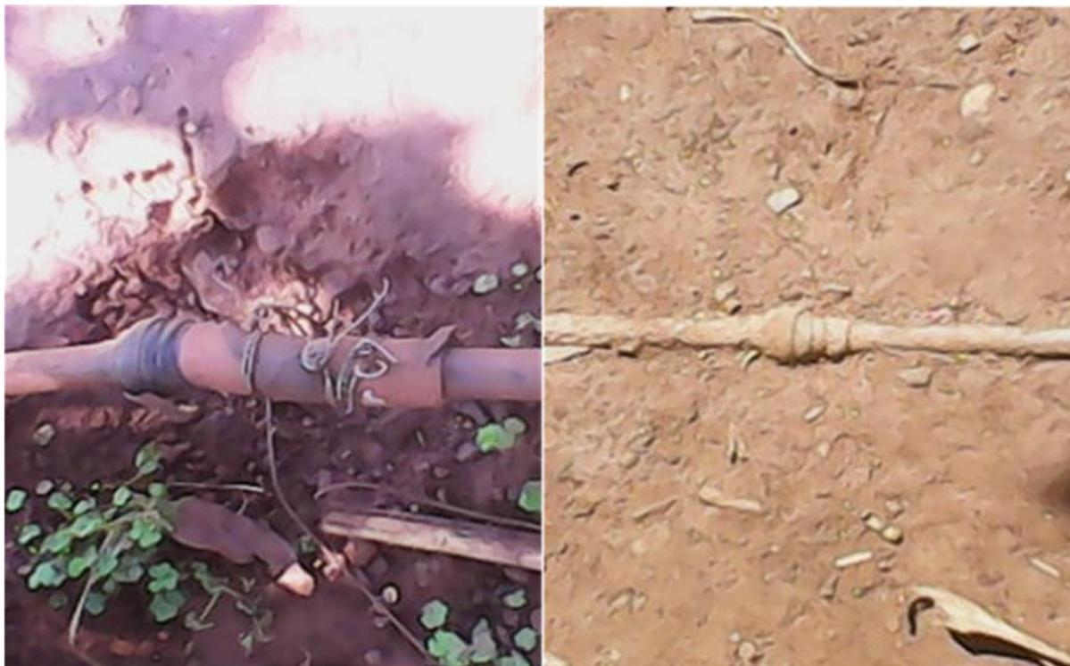
Plate 3: Two leaking pipes identified along service connections in Makusha residential area
