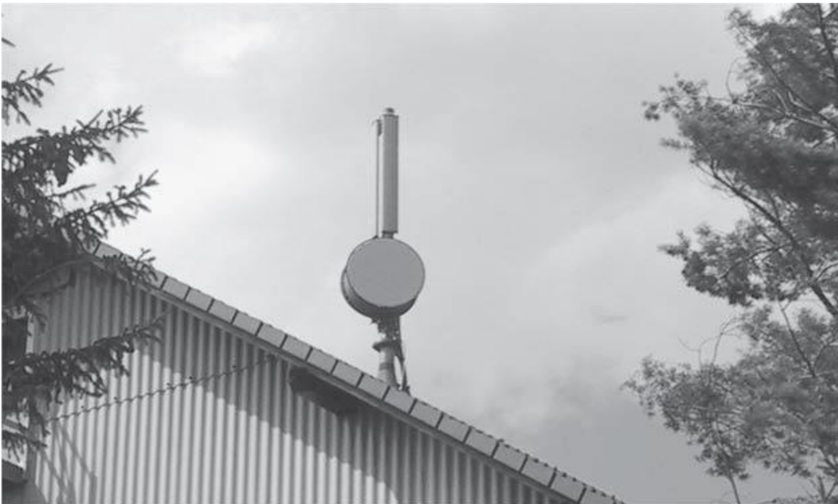
Fig 1.0 A typical antenna of a GSM base station. The optional microwave directional antenna (round antenna at the bottom of the mast) connects the base station with the GSM network [4].
