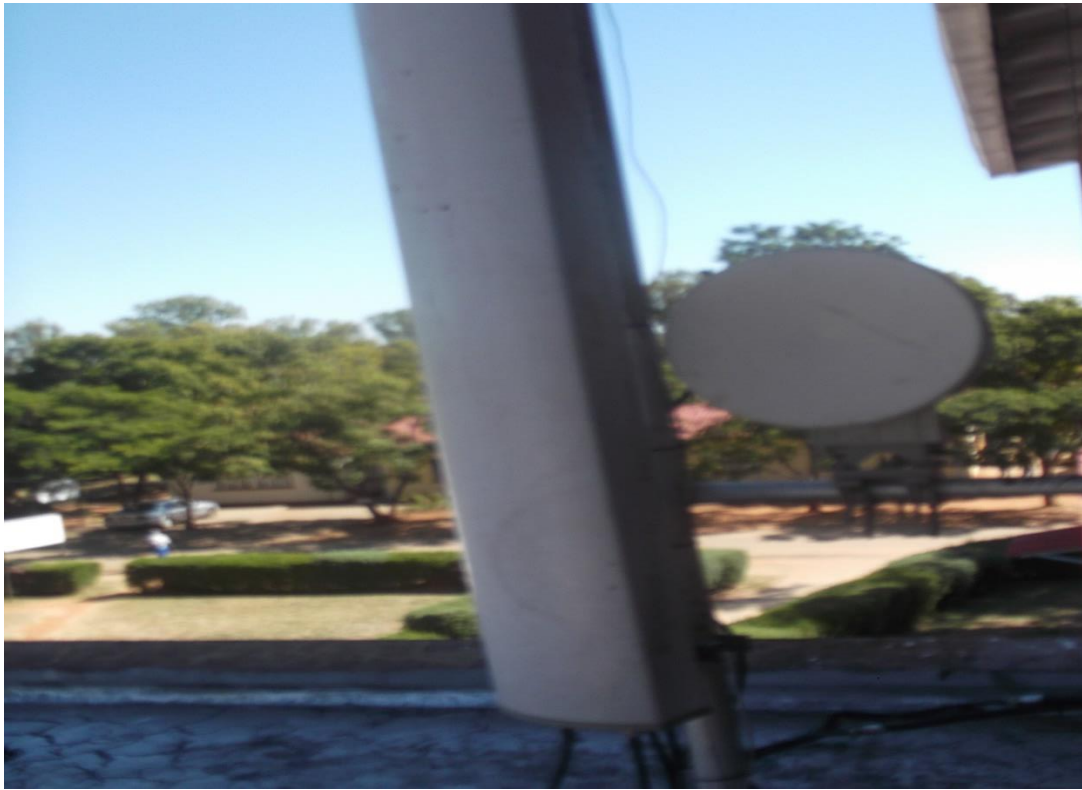
Fig 5.6 Microwave and GSM antennas
