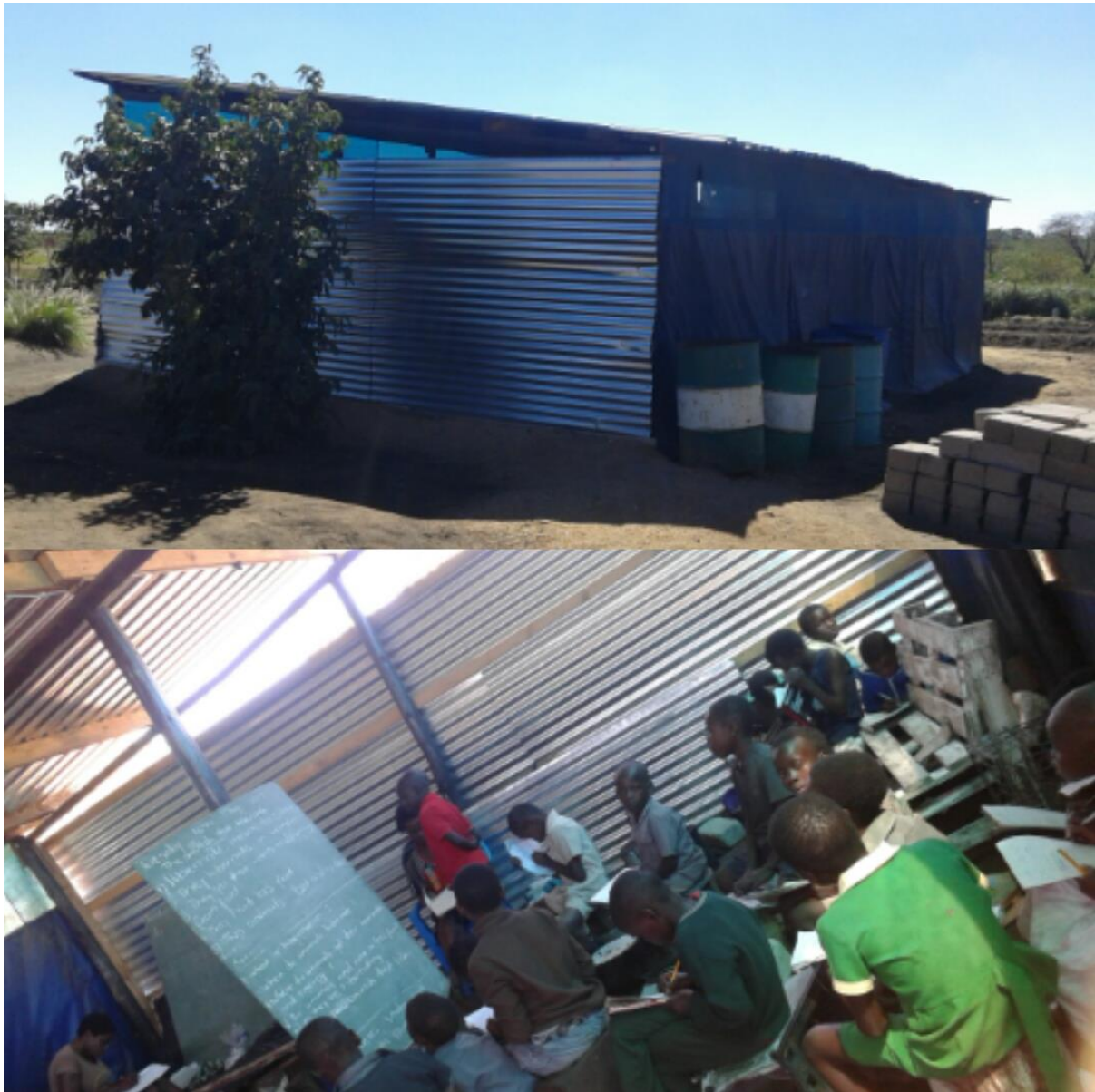
Plate 1: Interior and exterior of a classroom which is also used a church
