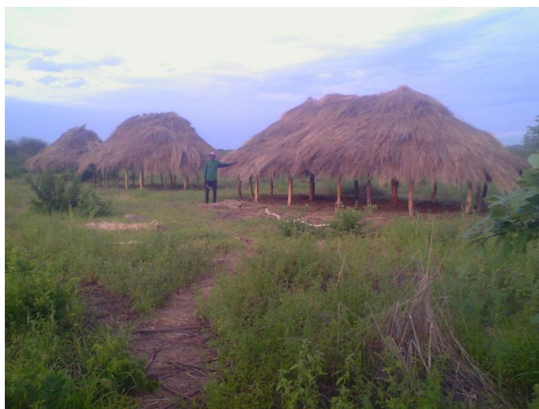
Figure 10: Infrastructure at one secondary school where children learn
