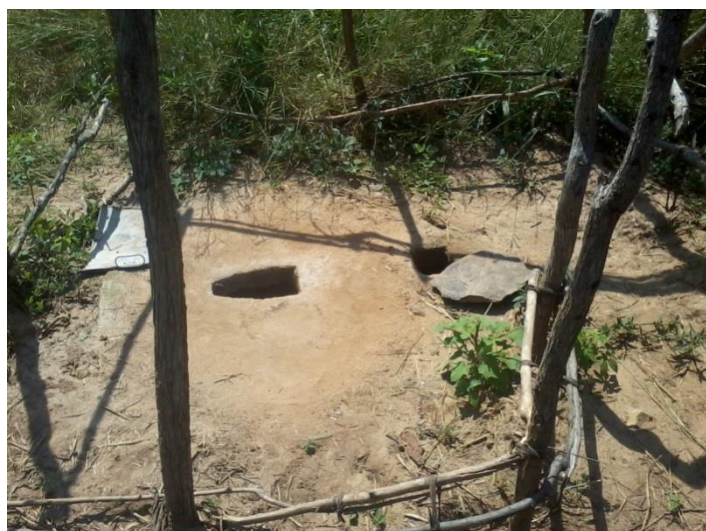
Figure 5: An incomplete toilet constructed through NGO assistance
